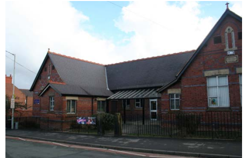
Slate Gable Roofs
