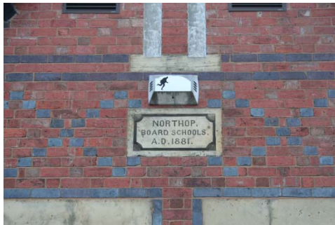
Patterned brickwork
